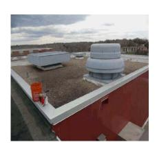
One (1) core cut revealed a steel decking. There is one (1) .25" layer of Dens-Deck, one (1) 3" layer of polyisocyanurate insulation board and one (1) layer of .50" wood fiber cover board. The membrane is a multiply BUR with a gravel surface.
