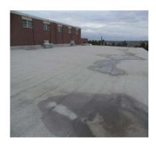
One (1) core cut revealed a precast concrete panel decking. There is a mopped vapor barrier, one (1) layer of 1.5" polyisocyanurate board and one (1) layer of .25" Dens-Deck cover board. The membrane is a two (2) ply modified bitumen with a granulated surfacing.
