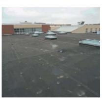
Core samples were taken on the C-1, C-2 and C-3 roof areas, each of which revealed the same type of roofing layers in place. The deck is poured in place gypsum. There is one (1) layer of 2" polyisocyanurate insulation board, one (1) layer of air-expanded polystyrene insulation, which appears to be part of a tapered insulation system, and a .5" layer of wood fiber cover board. The membrane is a fully-adhered, .060 mil Firestone EPDM.
